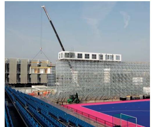
Above – cabins being craned into position on top of the grandstand using the largest cherry picker in the UK in terms of span
