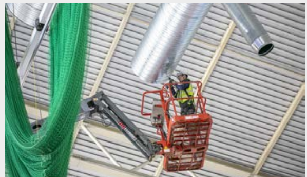
Boom lifter with operator wearing harness and restraint
