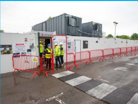
Crossing point with access gates
