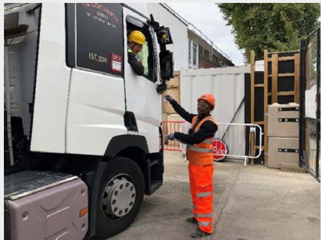
Traffic marshal checking driver information upon arrival to site
