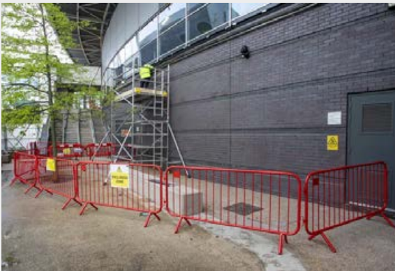
Robust exclusion zone formed around mobile tower works
