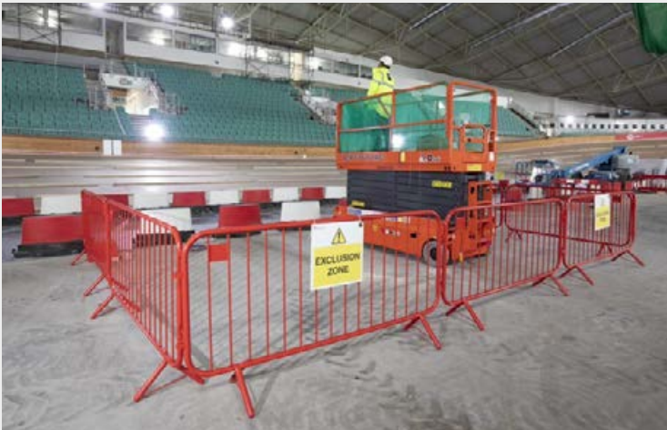
Scissor lift MEWP with robust exclusion zone
