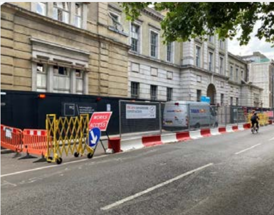
Segregated vehicle pit lane
