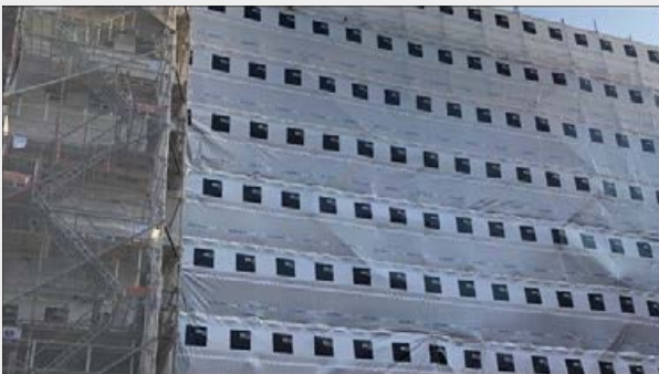
External scaffolding with full-height monoflex / containment netting
