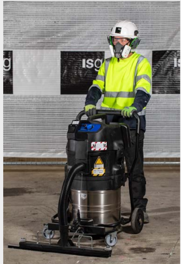
Clean-up operations with vacuum cleaner
