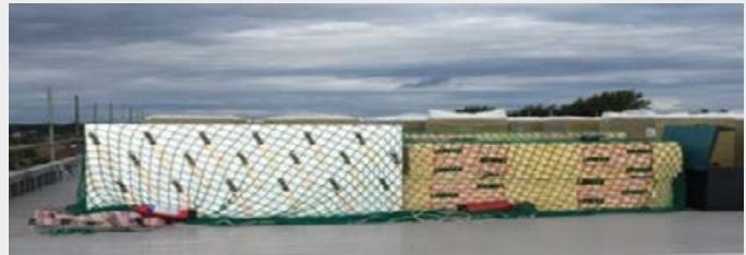
Lightweight materials secured at roof level with containment netting
