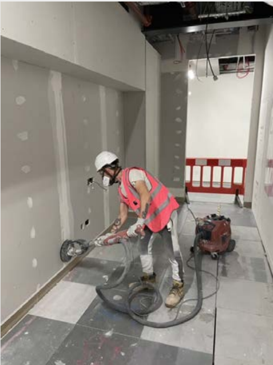
'M' class dust extraction in use
