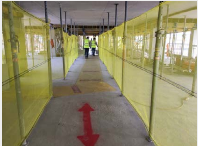
Internal / external access routes with anti-slip matting and clear directions
