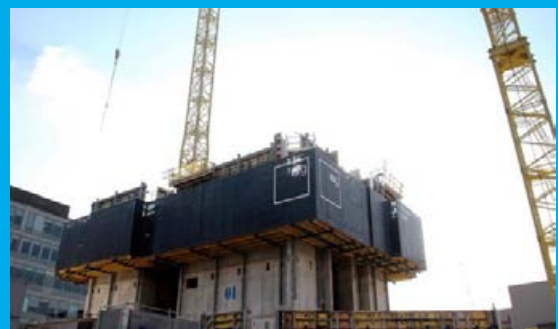
Safe screen system utilised to eliminate work at height
