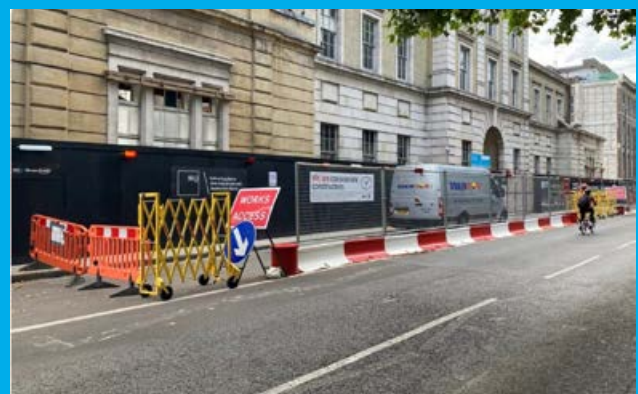
Pit lane providing segregation
