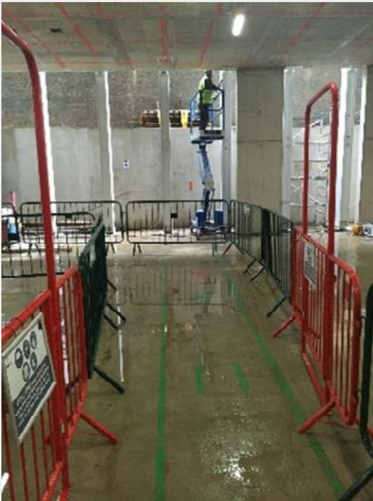
Internal access route
