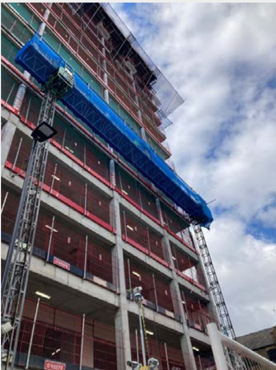
Mast climber with robust safety netting
