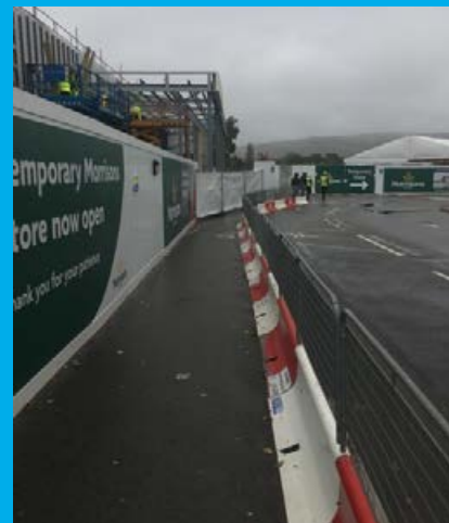
Pit lane providing segregation
