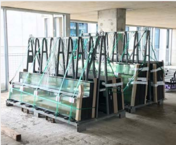
Glazing secured to stillage with individual banding
