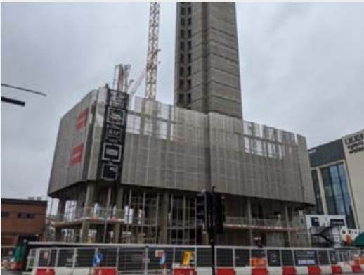
Safe screen utilised to eliminate falling objects
