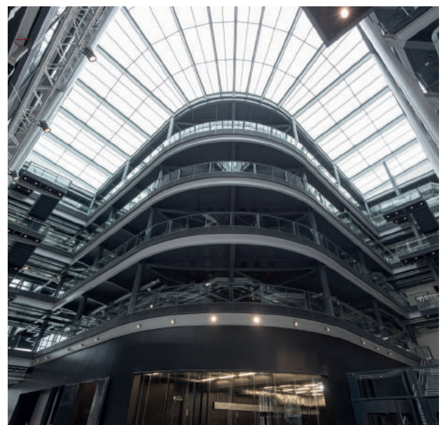
3 Central Square, Cardiff, UK – on target to achieve BREEAM 'Outstanding'
