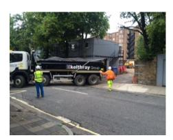
As vehicles leave the site they are cleaned by the use of a wheel wash facility to ensure that the local roads and surrounding areas are kept clean. The roads will also continue to be regularly cleaned so that there is no build up of earth and debris.
