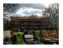
The concrete frame to the Art building is progressing well. The 2<sup>nd</sup> floor slab is currently being installed, with the ground floor & first floor walls and columns completed between March through to the start of April.
