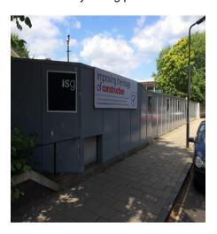
We have completed the hoarding installation to the perimeters making the site secure. We have also installed our 1<sup>st</sup> stage temporary offices and welfare facilities so as to afford us the time to get the ground prepared and available for the installation of the main accommodation block along the Loudoun Road elevation.
